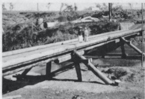
Coolabine Creek spider bridge, 1936. It was replaced by a wooden bridge in 1939 and the high-level concrete Houston Bridge in 1964.
