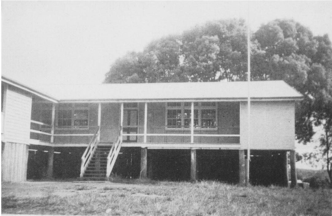
"New Section" Classrooms of Miss Roberts & Mr J Coyne
