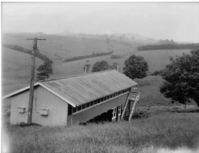
Manual Training & Domestic Science Building at the Maleny State School C1950
