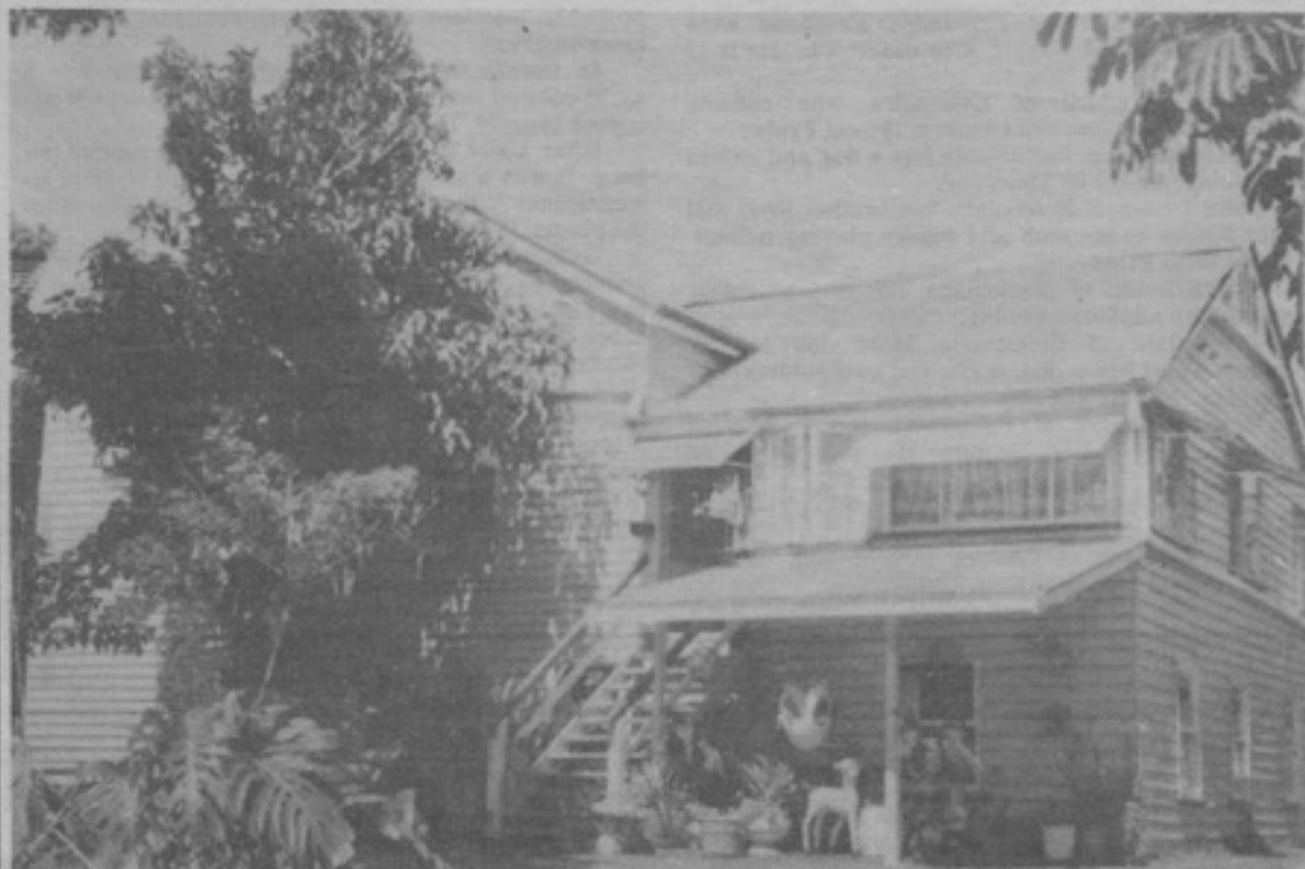
● ABOVE: The home of Eric and Ethel Howard, Maleny Road, as it is today. Part of the house came from Beerburrum Soldiers' Settlement.
