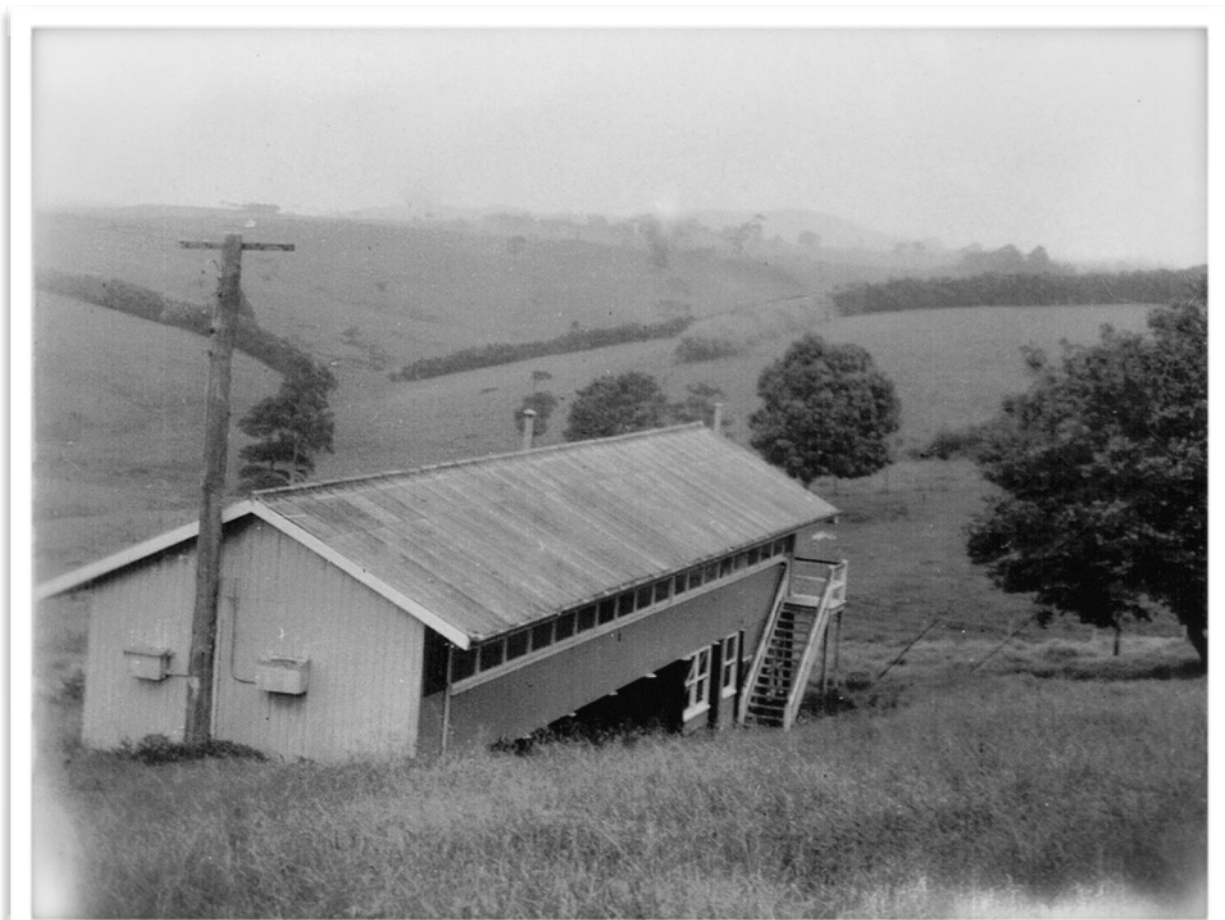
Manual Training & Domestic Science Building at the back of the Maleny School grounds in Cedar St
